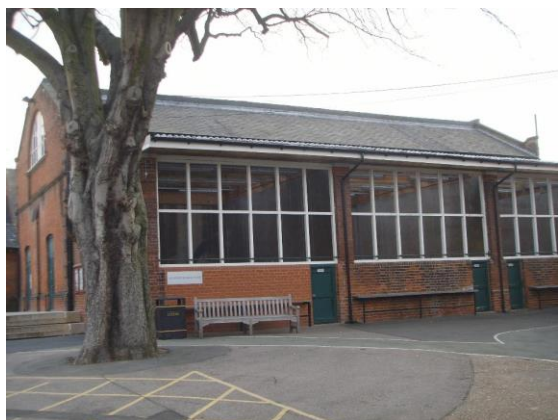
The 1905 small courts
